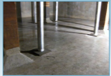
The Clearwell restoration project was completed last fall. The Clearwell, originally constructed in 1922, provides finished water storage. This aging tank was resealed and reinforced to allow for continued use.
