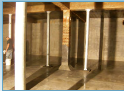
The Clearwell restoration project was completed last fall. The Clearwell, originally constructed in 1922, provides finished water storage. This aging tank was resealed and reinforced to allow for continued use.
