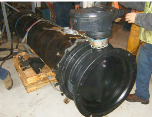
The new valve and pipe section being assembled prior to installation.
