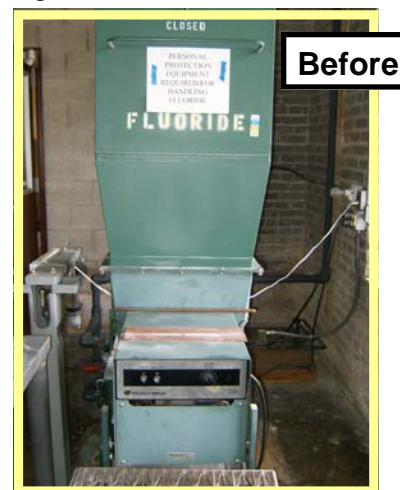
The twenty year old Fluoride Feeder was replaced, through a grant from the Michigan Dept. of Community Health
