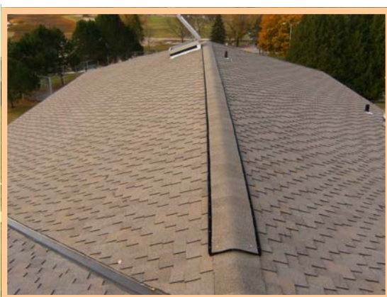
The Water Plant roof replacement was a capital improvement project in the fall of 2010. The surface was resheathed and new shingles applied.
